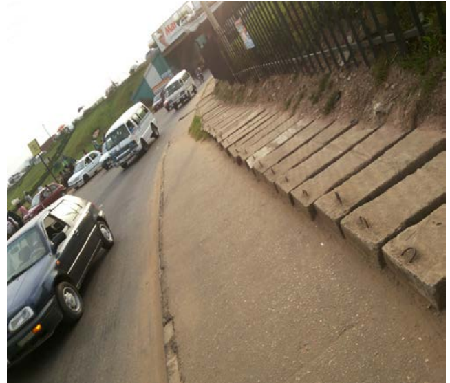
Plate 5: Restored condition of the rotary drainage
